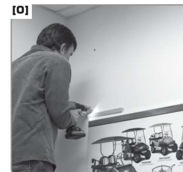
O] Remove Header and install Wall Anchors. • Replace Header and temporarily install top 2 screws. **DO NOT FULLY TIGHTEN**
