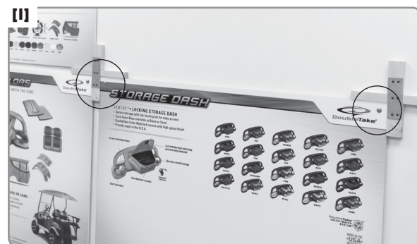
I] Use a Screw and Washer to TEMPORARILY attach the Panel in both top corners only. **DO NOT FULLY TIGHTEN**
