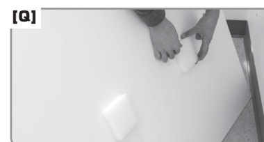
Q] Attach Plank Foam (x2) to the back of each Panel & Header, approximately at each third, to help support Panel centers.
