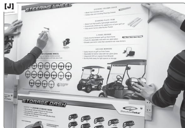
J] ** 2-PERSON JOB** Place the Top Panel onto the Install Jigs. Make sure the Jigs are snug and mark all 4 mounting holes for Top Panel.
