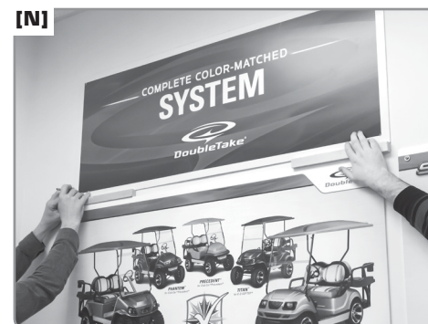
N] ** 2-PERSON JOB** Place the Header onto the 1" tall wood spacers (taken from Jigs in (K) above). • Align the edge of Header with the center line marked in (M) above. Mark the mounting locations. — NOTE: make sure to use the exact Header to be installed to mark hole locations, as the positions can vary since they are hand-drilled.
